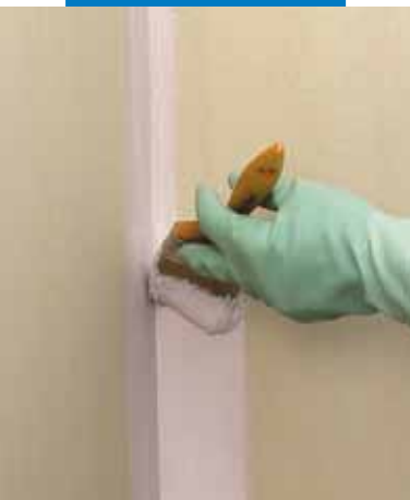
Applying Mapegum WPS with a brush
